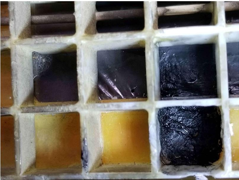
After cleanup. The exposed strands in the bottom square will get a little more grease to insure a seal against oxidation.
